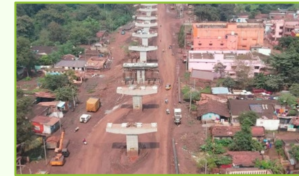
FLYOVER PROJECT - J ODA, ODISHA
