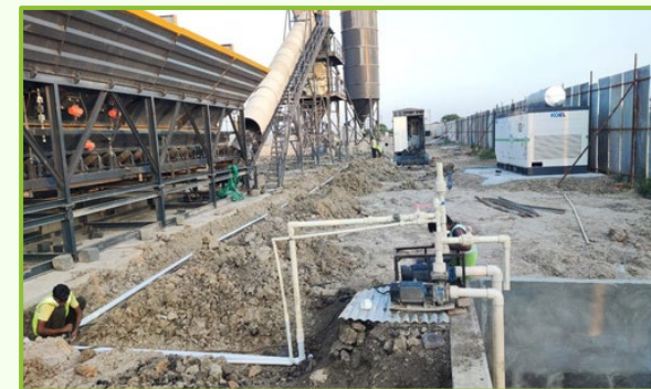
ROAD CONSTRUCTION - MBSIRDA, GUJARAT
