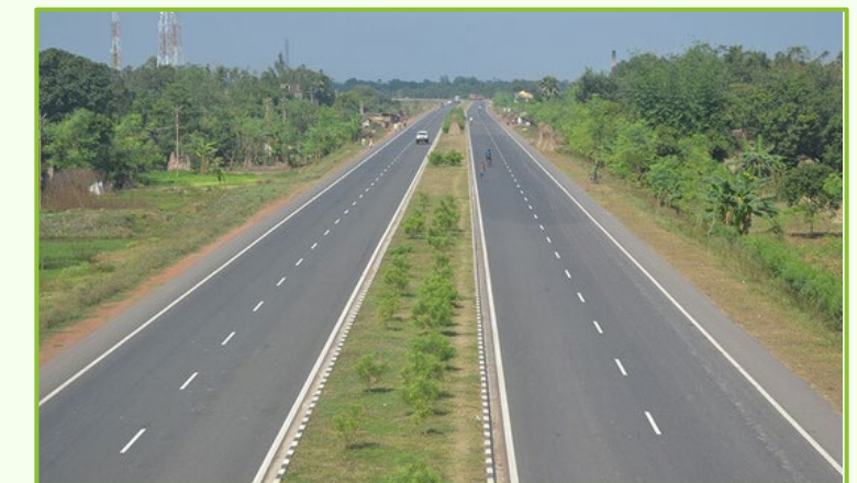
ROAD & STRUCTURE WORK - JETPUR SOMNATH ROAD PROJECT, GUJ ARAT
