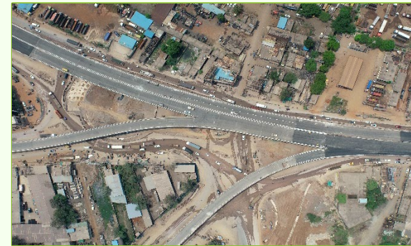
FLYOVER AND JUNCTION DEVELOPMENT - RAIPUR, CHHATTISGARH
