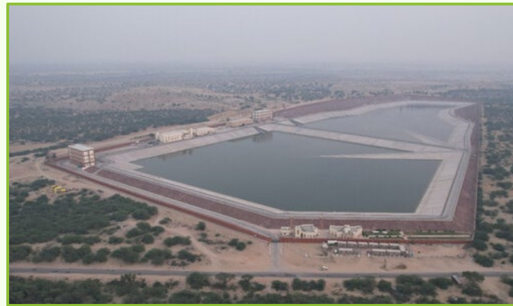
WATER RESERVOIR - NACHNA, RAJ ASTHAN
