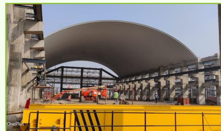
CAUSTIC SODA PLANT - DAHEJ, GUJARAT
