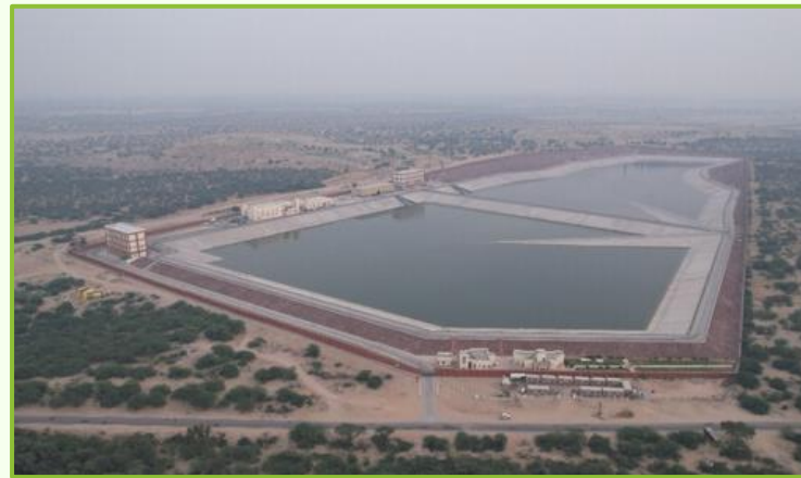
WATER RESERVOIR - NACHNA, RAJASTHAN
