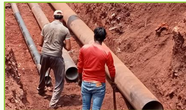
WATER SUPPLY - JODA AND CHAMPUA, ODISHA
