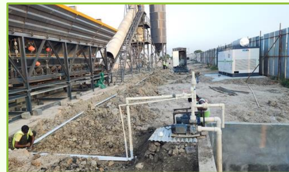
ROAD CONSTRUCTION - MBSIRDA, GUJARAT
