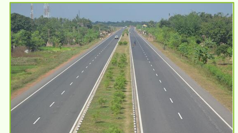
ROAD & STRUCTURE WORK - JETPUR SOMNATH ROAD PROJECT, GUJARAT
