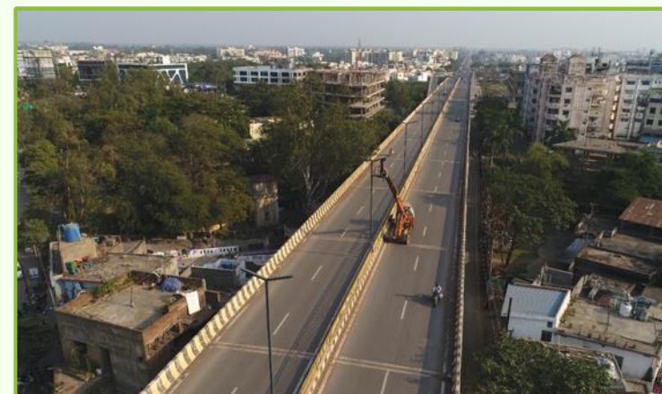
CONSTRUCTION OF FOUR LANE ROAD & FLYOVER - RAIPUR, CHHATTISGARH
